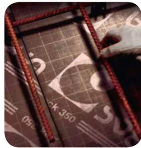
Convenient to place chairs and for rebar placement.
